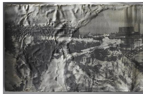
Fig. 2. Damage following the varnish removal and attempted removal from galvanized sheet metal: extensive staining ( top ); varnish present on area of extreme mechanical damage ( top center ); extensive losses to emulsion and support, severe staining ( bottom center ); and planar deformations ( bottom )
