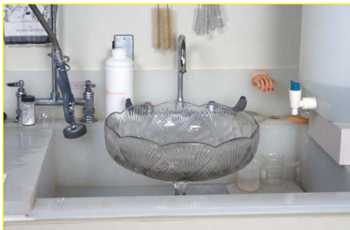
Figure 7. Polypropylene sink, with sprayer on the left, deionized water tank on the right.
